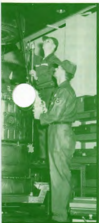
N-2 compressor on a J-75-19W.
